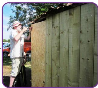
The base plate and about half the top plate are now renewed, and jointed into the fabric: two main posts are replaced, and the rest mended with half-lapped timber. The north wall has new cladding, and what is still usable from there will be used on the
